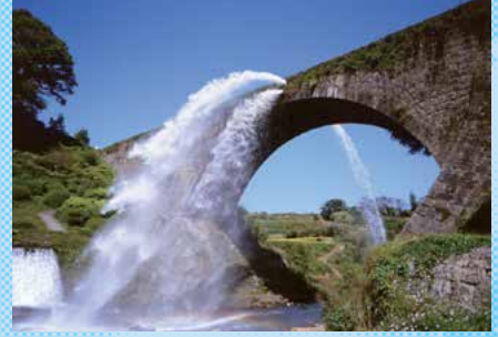
The Tsujunkyo Bridge is the only arched stone aqueduct bridge equipped with a water discharge function.
