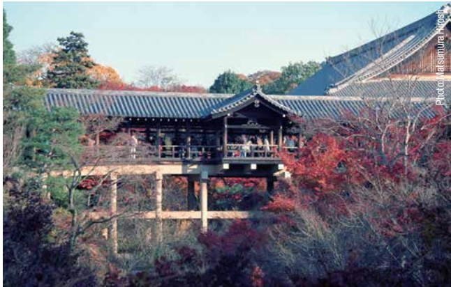
The Tsutenkyo Bridge at Tofukuji Temple in Kyoto City
